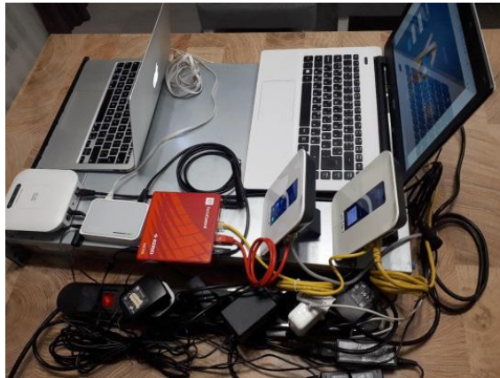
Figure 3. A practical realization of presented IT network with UTMs
